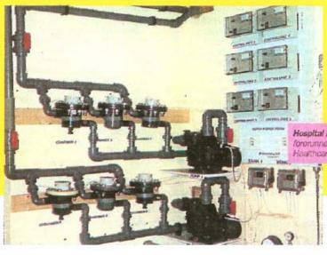
monitoring facilities and integration to computer management systems using the latest innovative technologies. It will be low cost, practical, environmentally sound and automatically release enough copper and silver ions to kill micro organisms whilst not exceeding the permitted levels of silver and copper within the ionised water.
